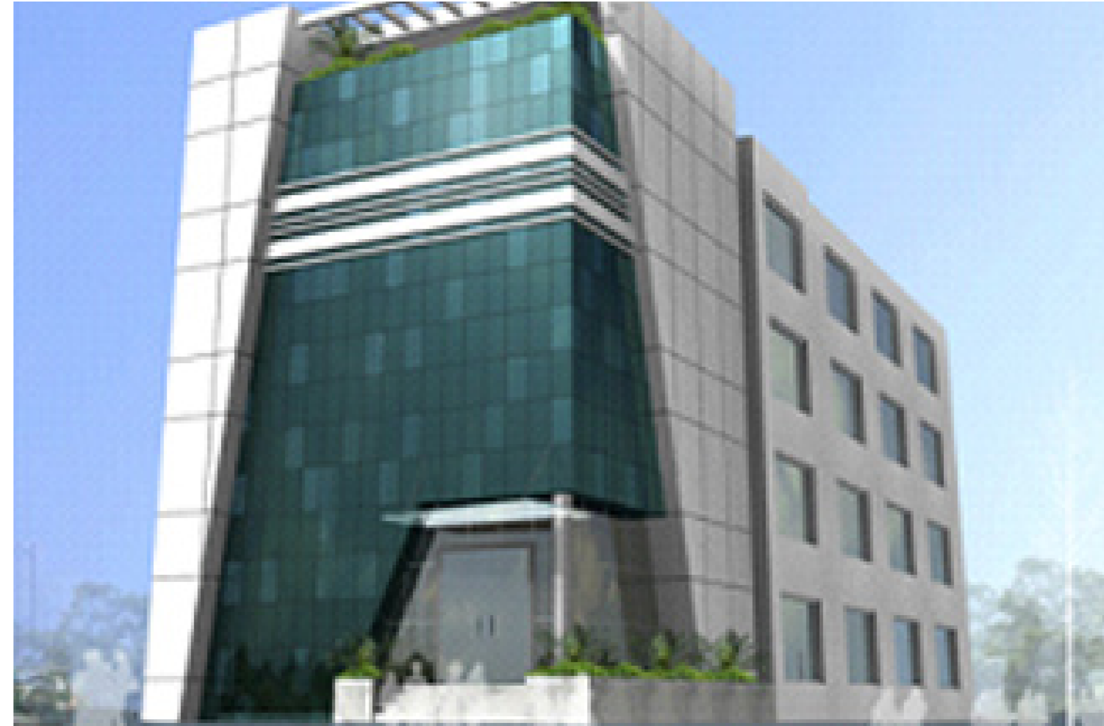
C-129, Sector 2 14,500 square feet.
